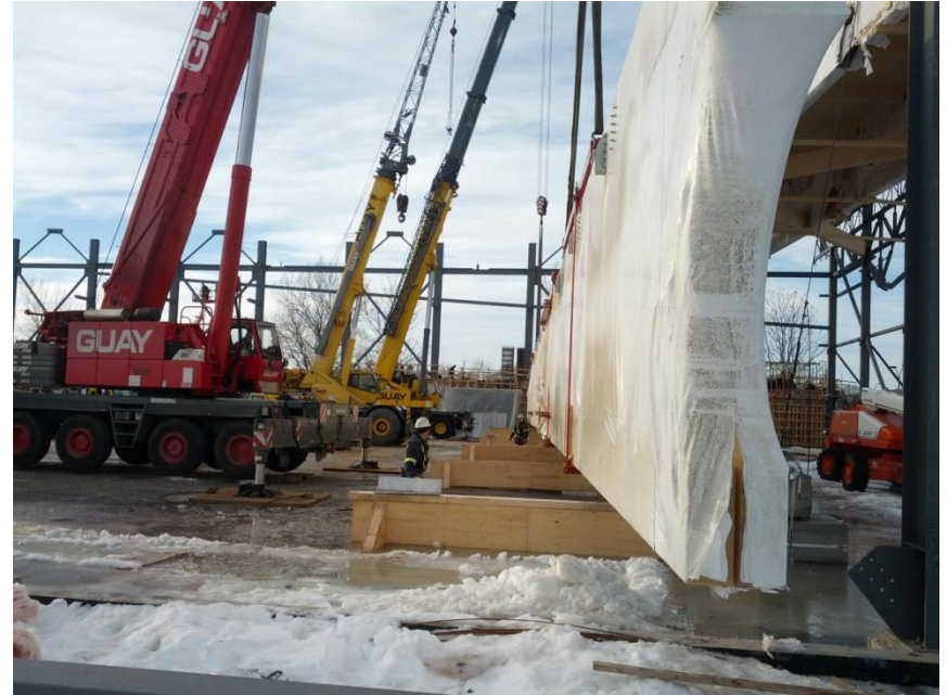
(2) Beam flipped up vertically
