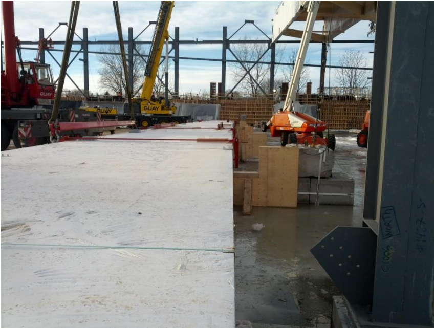
(1) Assembled flat on supports
